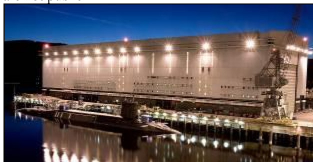
The Shiplift building with Vanguard-class submarine alongside on the adjacent 12 berth.
