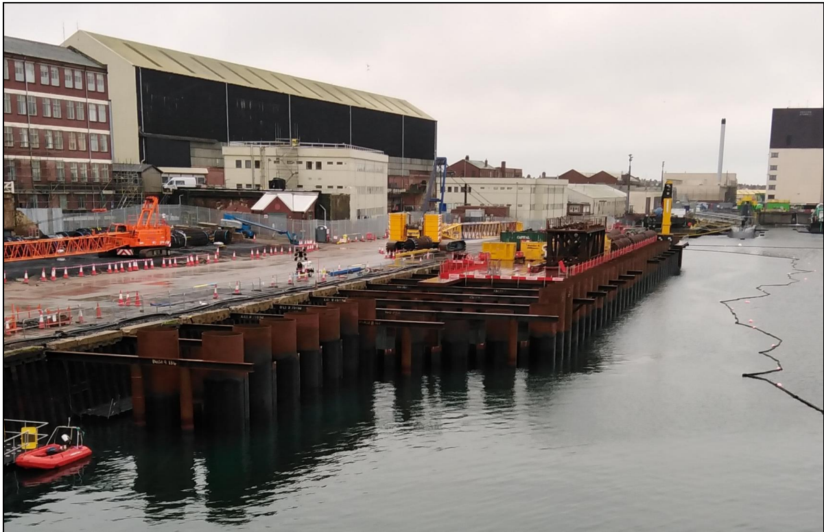
Progress on the New Wet Dock Quay – HMS ANSON in the background right
