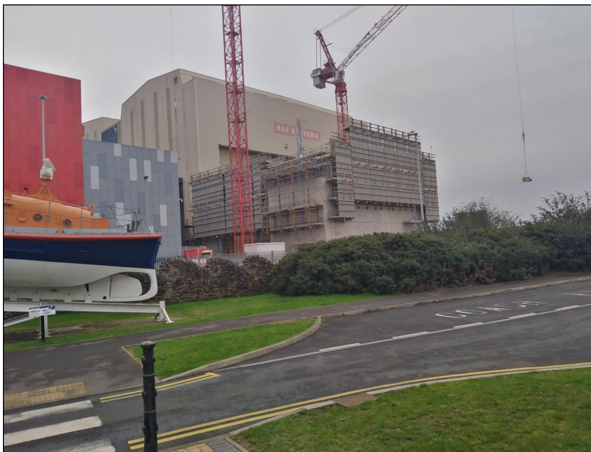
Still Growing – the Devonshire Dock Hall Extension
