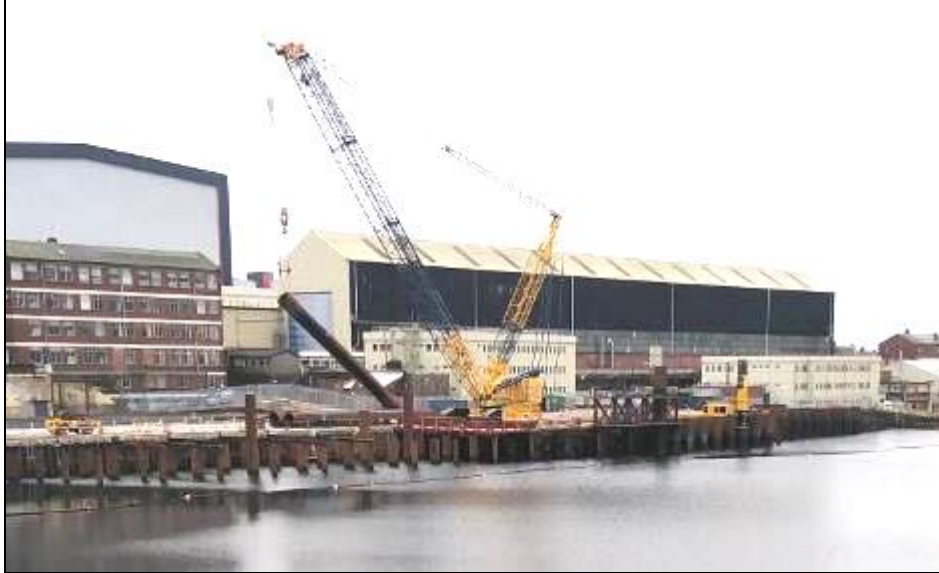
Lifting one of the piles before placing in position and driving into the floor of Devonshire Dock
