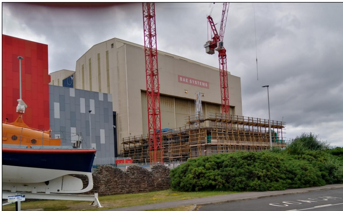
(1) Modifications to the Devonshire Dock Hall Entrance Under Construction (as viewed from the Dock Museum)
