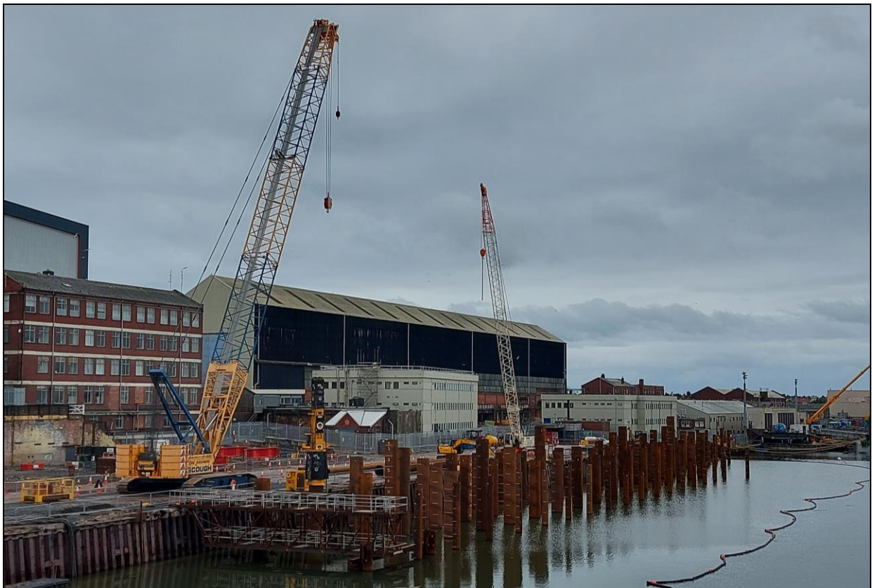
Progress on the Wet Dock Quay piling work 26 th June 2021
