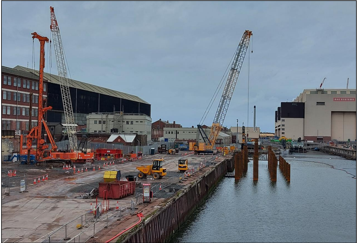
(3) Early Stages of the New Wet Dock Quay Piling work
